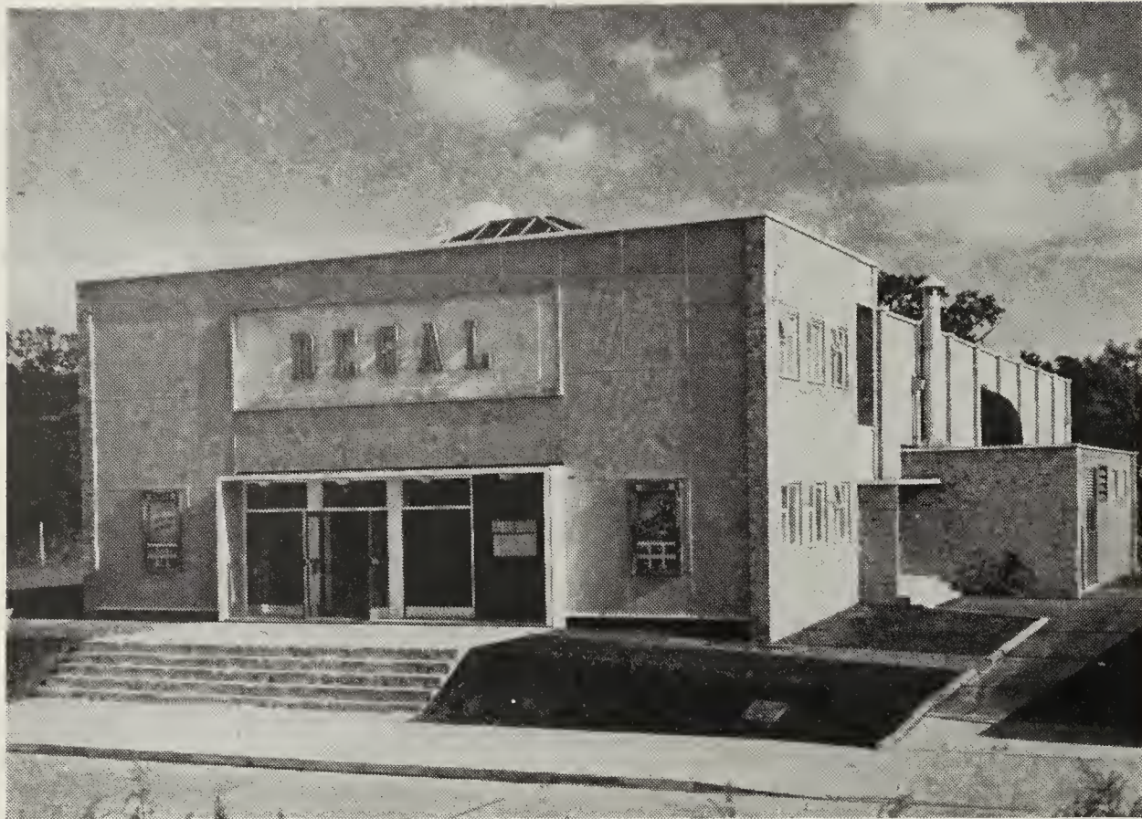
On the left: A view of the Regal, Harlow New Town, Essex, England. The frontage is so constructed that it can easily be torn down and replaced when the building reverts to its planned role as a factory. Above: The spacious projection room equipped by RCA with Ross projectors, Monarc arc-lamps, and Westinghouse rectifiers.
